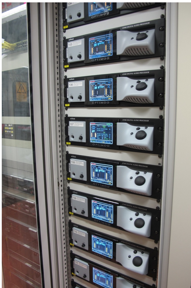
Rack with OPTIMODs for WDR2 in the MCR
